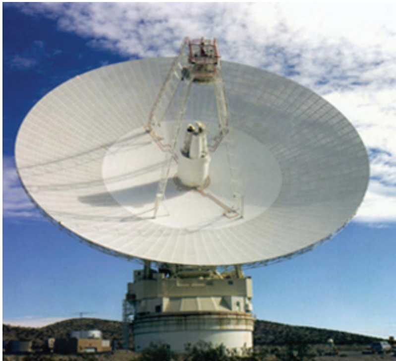
For over 40 years, the “Mars” 70-m Deep Space Network antenna at Goldstone, California, has vigilantly listened for tiny signals from spacecraft that are billions of miles away.
